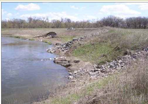
Same view as above but from farther upstream is the section of bank that gave way. (spring 2009)
