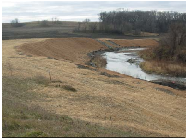
Same view, construction completed (October 2007)
