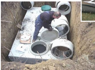
replacing a septic tank and drain field
