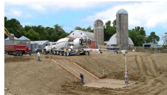
feedlot improvements under construction
