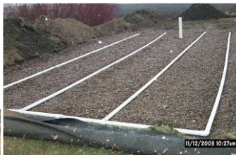
replacing a septic tank and drain field
